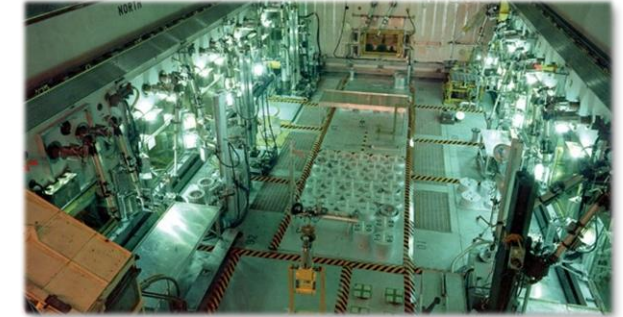
Hot Fuel Exam Facility
